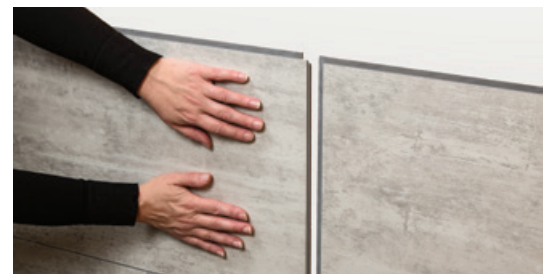
Lock tiles by sliding into joint
